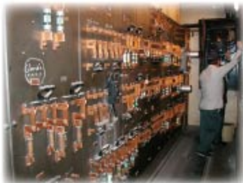
Recent service to an old switchboard
